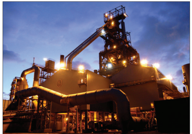
Port Talbot blast furnace © Corus
